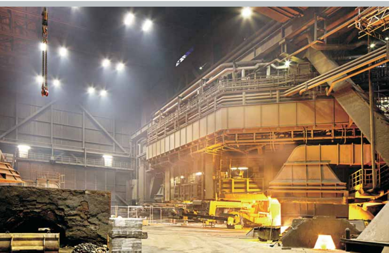
REVO Hallenbeleuchtung / REVO Hall lighting
